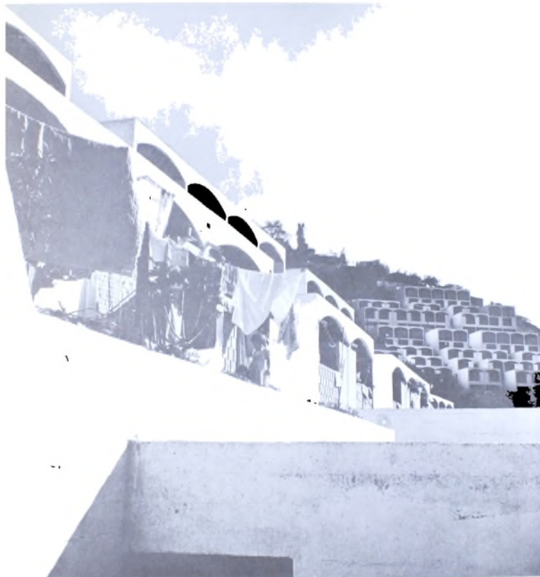
93. Roland Simounet: Cité de Recasement, Djennan-el-Hassan, Algeria.
