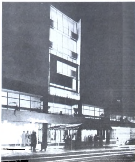
59. Architects' Co-Partnership: Bristol Hotel, Lagos, 1962.
