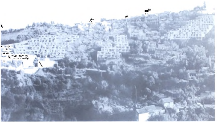
91. Roland Simounet: Cité de Recasement, Djennan-el-Hassan, Algeria
