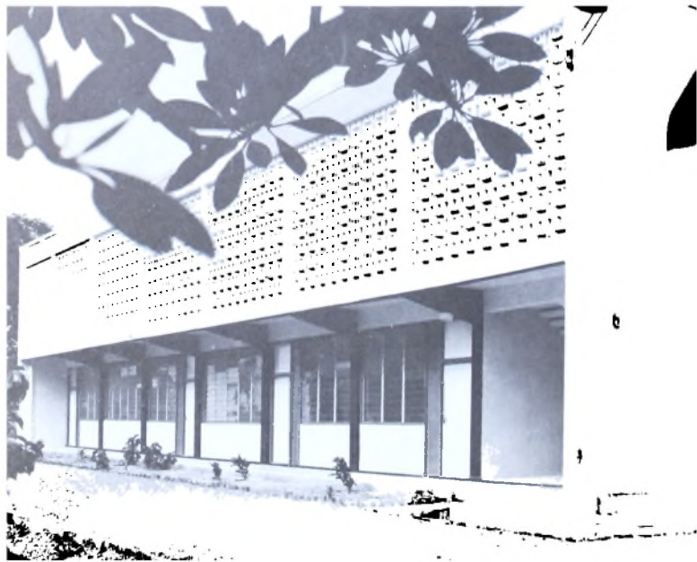
12. A. Ileanyi Ekwueme: Laboratory Building, St. Gregory's College, Lagos, Nigeria.
