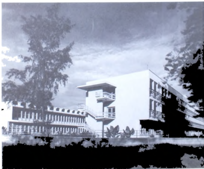
66. A. Itanyi Ekwueme: Hospital for Nigerian Railway Corporation, Ebute Metta, Lagos, Nigeria.
